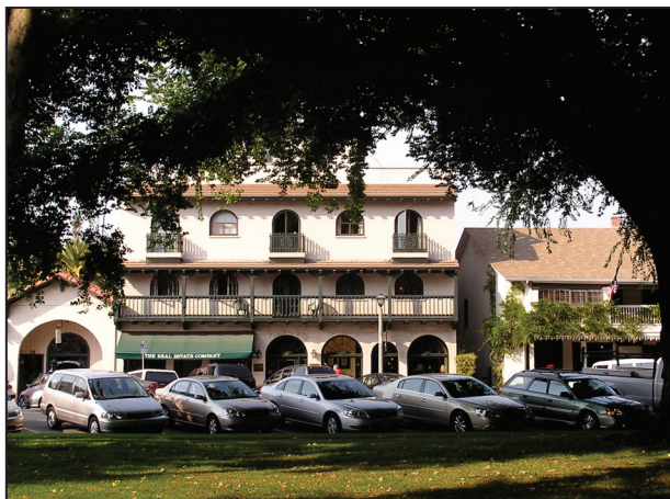
The Cuneo Apartments—A historic example of mixed use.
